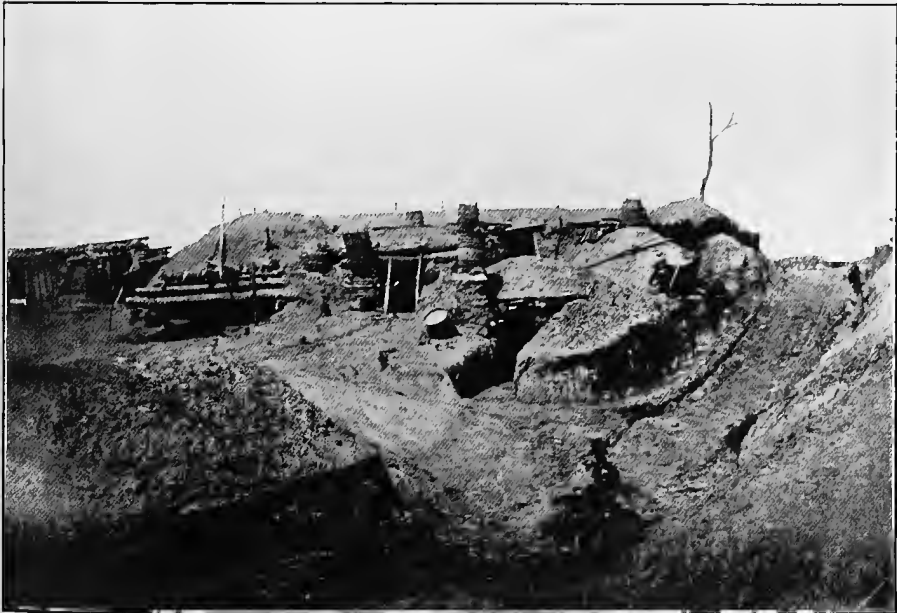
BOMB-PROOF HEADQUARTERS SEVENTH REGIMENT R. I. VOLS. IN FORT SEDGWICK. TUB AT LEFT OF ENTRANCE.
